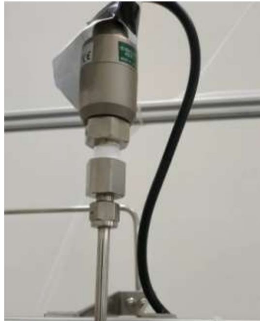
Figure 5. Installation of 4 Pressure Transmitter on Methanol Testplant
