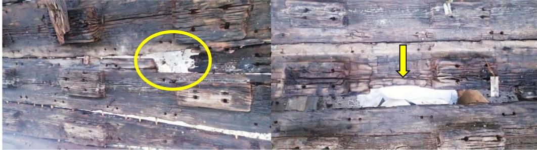
**Figure 14.** Damaged Planks Caused by a Flaking Process
