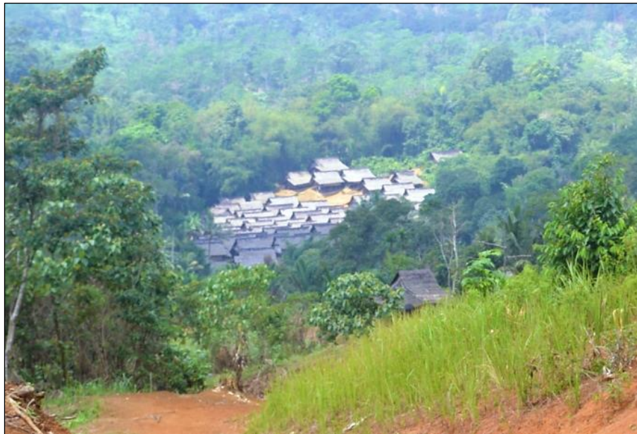
Figure 5. The settlement of the Baduy Dalam community in Cikeusik captured from afar (Source: Nurrochsyam, 2016 )
