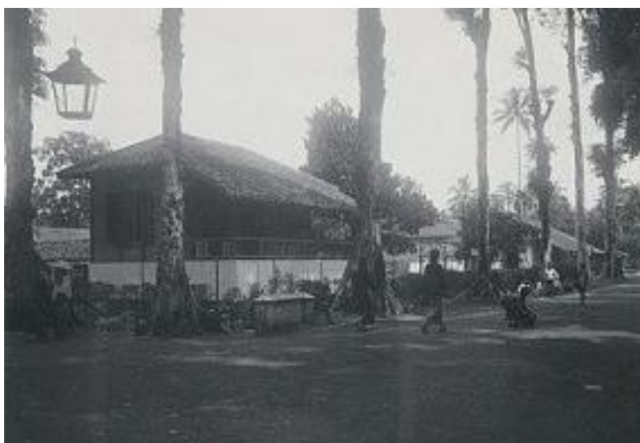
Figure 3. Military Hospital in Cilacap (Source: https://historicalhospitals.com/military-hospitals/garrison-hospital-cilacap/ ).
